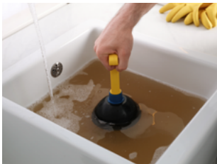
Clearing blocked sinks, basins, and showers
