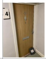
9.1, 9.5, 9.16 During the previous fire risk assessment, several doors within the caretaker rooms could not be closed/locked at the time of the assessment. It was confirmed by WCHG that this action has been completed by HG Maintenance It was confirmed that the doors had been repaired. Completion date 10/09/2024.
