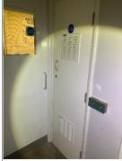
On the escape side of the electromagnetically secured laundry door, both release devices are identical, these being 'push button to exit' devices. Neither of the buttons is labelled as the override.
