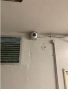
CCTV equipment was observed in the common areas, with the associated equipment located in the main electrical intake cupboard.
