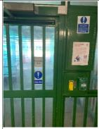
Where electromagnetically secured doors were observed as fitted on the premises (e.g. main entrance door/laundry corridor door), these were provided with suitable overrides on the escape side.
