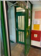
The 'main entrance' final exit from the lift lobby and the exit at the base of the staircase serving all floors discharge within 1.8m of each other and the surrounding glazing does not appear to be fire resisting. Although this does not meet the requirements of current guidance, this has been accepted on the basis that robust control measures are in place to ensure these areas remain sterile at all times, therefore the probability of a fire beginning in either of these areas is negligible.
