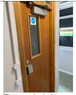
Electromechanically secured doors separate the staircase from the corridors serving flats and these require fob access in the direction towards the flats. In the direction of escape, a suitable push pad device is provided leading into the stair.
