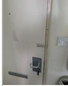
The fastenings on the internal side of the existing flat entrance doors were key operated, however our assessor has observed the new flat entrance doors to be installed (which were already in place in Brownley Court and Hollyhedge Court) and these were provided with thumb turn devices.
