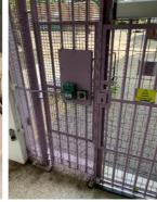
8.18-8.19 As part of WCHG's standard responses, they have confirmed that due to most FRAs raising a finding, WCHG had engaged with Tech Sol and confirmed that doors fail safe/open upon a fire alarm activation or loss of electricity, and that break glass points are installed as a back up should the push to exit button fail.
