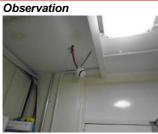
The above photograph shows a smoke detector in the caretaker's area has been displaced and may be damaged. A damaged smoke detector may not give an early warning of fire thereby placing persons at risk of harm.
