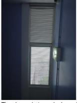
The above photograph shows the permanently open vent at the top of the single stairway. The lobbies to the flats also have a permanent vent. The stairway and the flat lobbies are separated by the lift lobby. The current provision for smoke ventilation is acceptable at this time.
