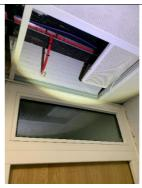
False ceiling tiles were installed in the common areas. A number of areas above the false ceilings were inspected and it was observed that fire stopping works had been carried out in these areas, including where services passed into flats and above lobby doors.
