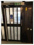
Where electromagnetically secured doors are installed within the premises (e.g. final exits, external exit from forecourt, laundry), these were observed to be accompanied by suitable green box emergency overrides.
