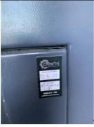
In the bin room on the ground floor, the bin in use is located adjacent to a lid that has a fusible link and closes should a fire occur within the bin to prevent fire spread up the chute. In the refuse chute rooms, metal chutes are provided which are self-closing. The fusible link is checked annually by an appointed contractor, with labels fitted to bin equipment indicating that this was last carried out on 19/04/2022.
