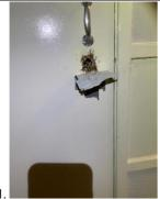
Several riser cupboard doors could not be locked shut at the time of the assessment, detailed as follows:
