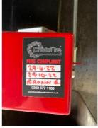
In the externally accessed bin room on the ground floor, the bin in use is located adjacent to a lid that has a fusible link and closes should a fire occur within the bin, in order to prevent fire spread up the chute. The fusible link is checked six monthly by an appointed contractor, with a label indicating that this was last carried out on 29/04/2022.
