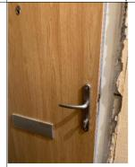
The new fire doors that are being fitted to flats have thumb turn type locking devices on their internal side.
