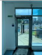
Several final exit doors from the building were electromagnetically secured and were accompanied by suitable green box emergency overrides. The same electromagnetically secured door and override arrangement is provided to the fire resisting doors which separate these two exits. It was previously confirmed that these doors are configured fail to the openable position on activation of the fire alarm system.
