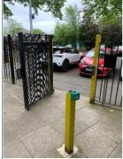
As previously recommended, the electromagnetically secured gate outside the main entrance has been provided with a green box emergency override on the escape side, enabling persons to proceed to a place of ultimate safety upon leaving the building.
