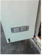
In the riser cupboards adjoining the open deck, metal grilles are located in the lower portion of doors. When shining a torch through the grille, our assessor was able to view the light passing through. Where there is inadequate protection of the adjoining open decks, persons passing the cupboards in order to escape may be placed at risk of harm.
