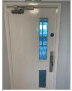
The access doors to all the open decks are fitted with electromechanical locks. They are provided with push pads or lever handles that allow them to be opened on the open deck side of the door without the use of a key.
