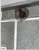
In the flats that were viewed during this and previous Fire Risk Assessments, it was confirmed that the ventilation arrangements for the kitchen and bathroom were located on the external wall onto the open deck and did not pass through any other compartmentation. The extraction passes out of the flats at high level, therefore does not affect persons escaping past. Extraction from the laundry was observed to lead directly to outside.
