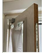
The resident of flat 47 (fourth floor) has removed the self-closing device to their entrance door. Where flat entrance doors along the single direction deck are not effectively self-closing, passing persons may be at risk of harm.
