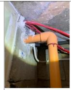
As recommended at the time of the previous fire risk assessment, the numerous fire alarm cable breaches identified has been sealed using appropriate fire stopping materials.
