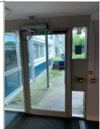
WCHG have previously confirmed that the electromagnetic locks within the premises are linked to the common fire alarm and conform to BS7273-4. Where electromagnetically secured doors within the building were observed (e.g. final exits and laundry door), these were accompanied by 'push button to exit' devices and green box overrides.
