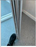
The inner refuse chute room door on the fourth floor is not effectively self-closing and this is due to the strip and seal coming loose. Where fire doors are not effectively self-closing and do not efficiently prevent the spread of products of combustion, persons may be placed at risk of harm.
