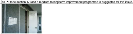
New fire doors have been fitted in various locations throughout the premises. This includes all the riser doors on the balconies where all the new fire doors have been provided with intumescent grills and are kept locked shut. All new fire doors have been fitted using three hinges, have intumescent strips and cold smoke seals. They are also provided with a suitable self-closing device or are kept lock shut and are suitably signed.
