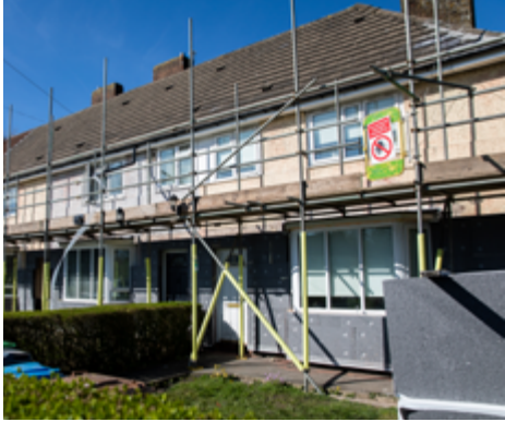
During the work
