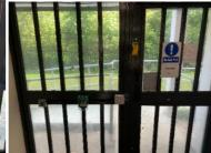
8.21 The emergency override on the escape side of the electromagnetically secured laundry door is now labelled as an override.
