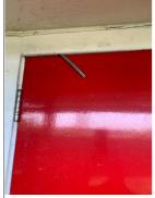
The strip and seal on the top edge of the electrical cupboard (fifth floor) was loose and appeared to be coming off. The service riser cupboard by flat 43 (fifth floor) was missing a strip and seal.
