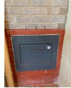
In the bin room on the ground floor, the bin in use is located adjacent to a lid that has a fusible link which enables the lid to selfclose over the bin should a fire occur. This is to prevent the fire, smoke and toxic gases spreading up the chute. The fusible link is checked annually by an appointed contractor and a label indicated that this was last carried out on 19/04/2022.
