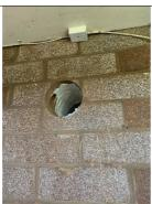
In the flats that were viewed during this and previous Fire Risk Assessments, it was confirmed that the ventilation arrangements for the kitchen and bathroom were located on the external wall onto the open deck and did not pass through any other compartmentation. The extraction passes out of the flats at high level, therefore does not affect persons escaping past. It was observed at the time of the assessment that vents were being lined with fire stopping materials.
