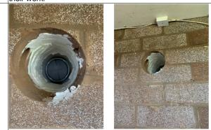
In the flats that were viewed during this and previous Fire Risk Assessments, it was confirmed that the ventilation arrangements for the kitchen and bathroom were located on the external wall onto the open deck and did not pass through any other compartmentation. The extraction passes out of the flats at high level, therefore does not affect persons escaping past. It was observed at the time of the assessment that vents were being lined with fire stopping materials.
