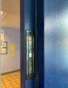
The front entrance door to the residential premises is electromagnetic, with an emergency override provided on the escape side. The same arrangement is present from the laundry back into the main entrance foyer.
