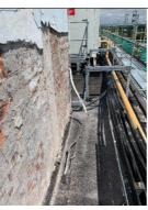
The lightning protection system for the building has currently been removed in preparation for the roof covering of the building to be replaced. Generally, where lightning protection systems are fitted, WCHG ensure that these are serviced annually by a competent person, with records held centrally.
