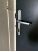
Adjudging by the provisions within the sample flats accessed, thumb turn type opening devices are fitted to the internal side of resident flat entrance doors
