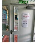
The main final exit door from the community room is thumb turn operated, with the rear exit being push bar operated.
